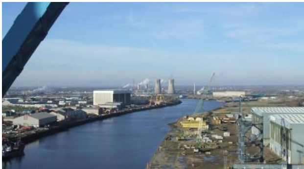
River Tees from the Transporter Bridge
