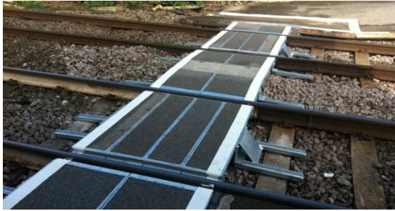
An example of boarding out a footpath; Stockton on Tees have had recent success with Network Rail.
